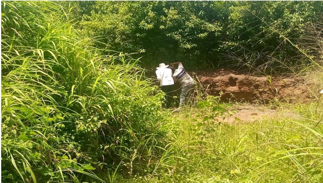
Excscivtion the borehole
