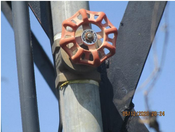
This 2” gate valve need replacement with ball valves. Electrical wiring faulty needs replacement for For the 2 sites.
