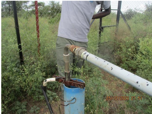
This 2” gate valve need replacement with ball valves. Electrical wiring faulty needs replacement for For the 2 sites.
