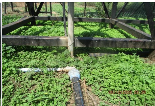
Reference point of connection from tank outlet. To The manifold and to the new pipe- line for leading To the water troughs.
