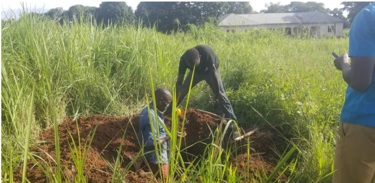
Excavation of the boreholes
