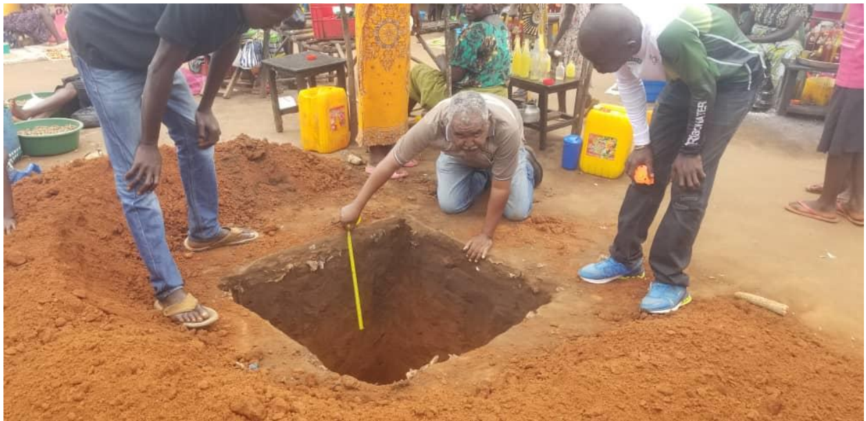
Excavation the borehole
