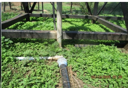
Reference point of connection from tank outlet. To The manifold and to the new pipe- line for leading To the water troughs.
