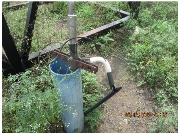
A conventional well head cover is required to Replace the clamps, needed for all the two sites.
