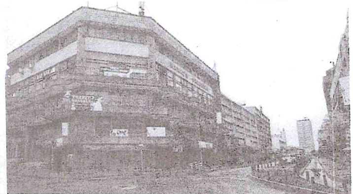
Closed shops on Luwum street on March 27 as a result of the lockdown
