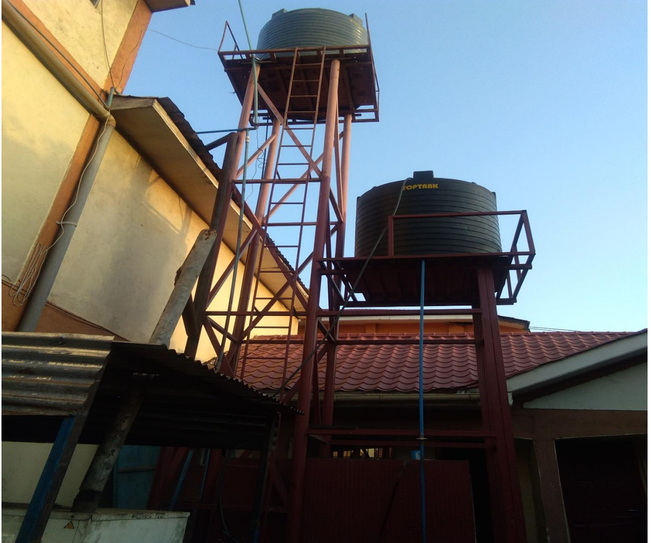
TWO BIG WATER TANKS FOR CONSTANT WATER SUPPLY TO THE OFFICES
